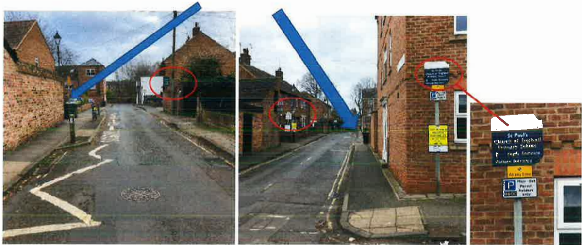
School keep clear zone and double yellow zone on Watson Terrace and Pupils entrance sign on junction with St Pauls Square
